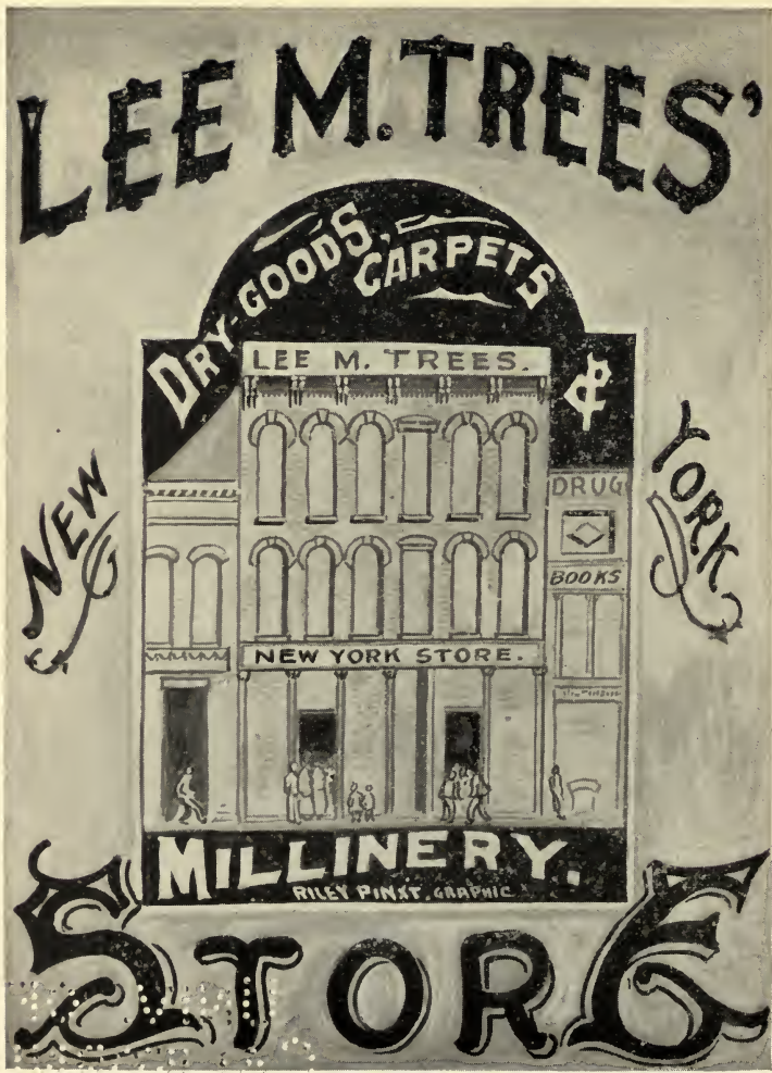
NEW YORK STORE SIGN AT ANDERSON
